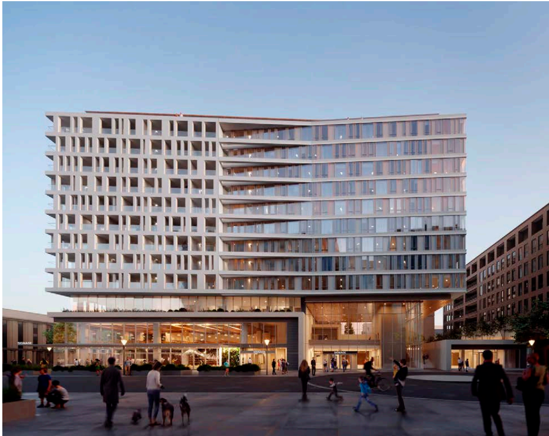
RESIDENTIAL CCIII VIEW FROM G STREET ROUNDABOUT
