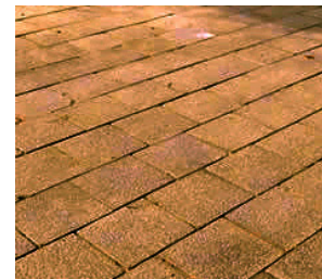
PAVING PRESSED CONCRETE PAVERS
