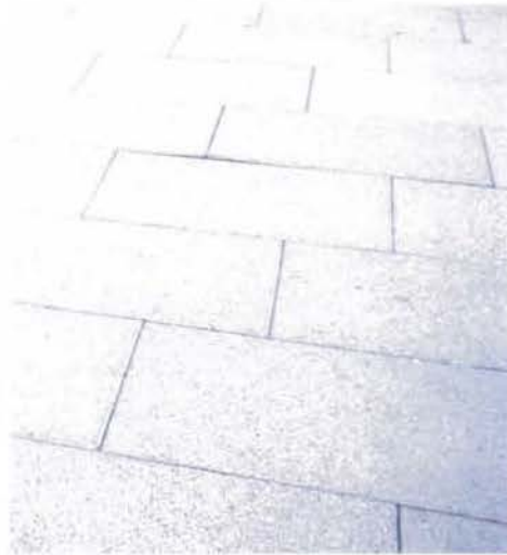
PAVING - 2'X3' PRESSED CONCRETE PAVER
