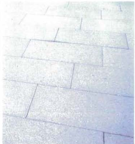
PAVING - 2'X3' PRESSED CONCRETE PAVER
