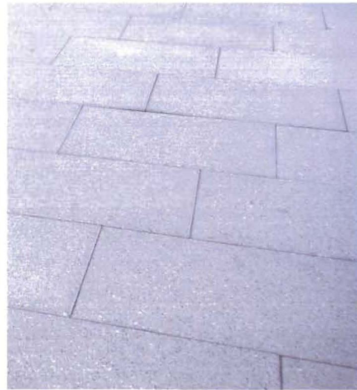
PAVING - 2'X3' PRESSED CONCRETE PAVER
