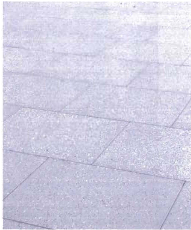
PAVING - 2'X3' PRESSED CONCRETE PAVER
