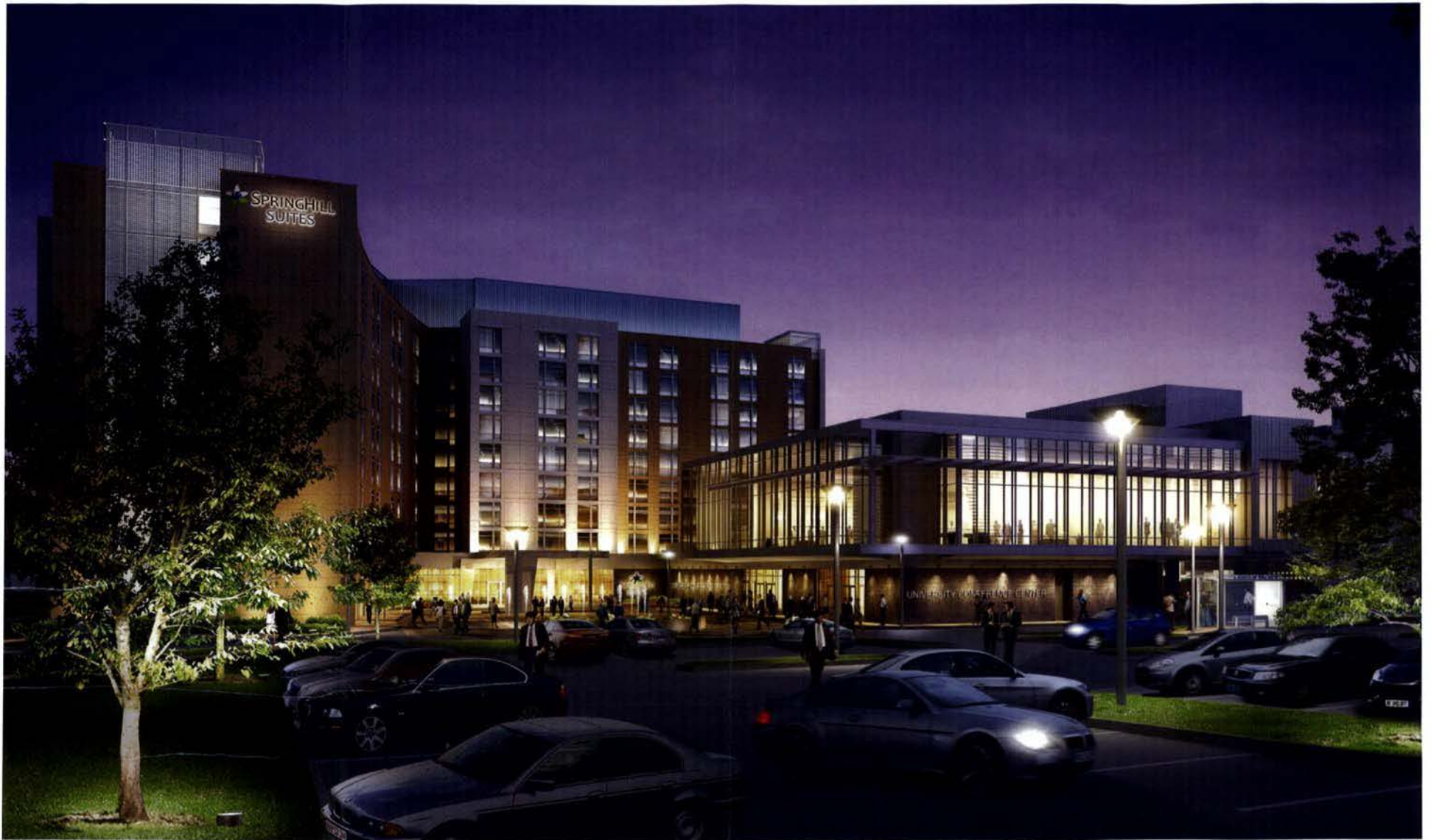
A-27 Approved Evening View of Main Entrance Michigan Avenue & Irving Street NE Mixed-Use Complex | Washington, D.C.
