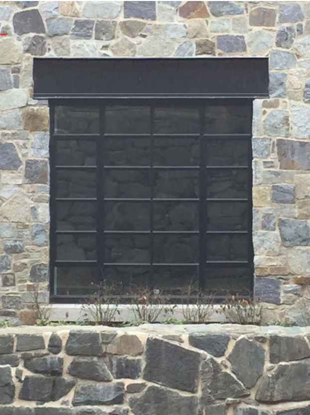
STEEL LINTEL DETAIL AT STONE BASE
