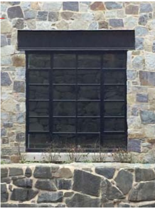
STEEL LINTEL DETAIL AT STONE BASE
