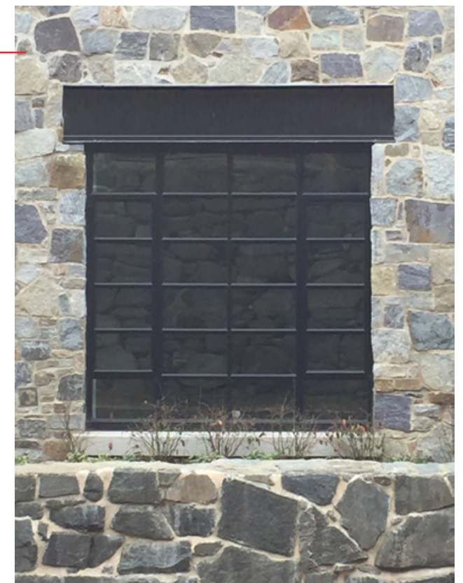
STEEL LINTEL DETAIL AT STONE BASE
