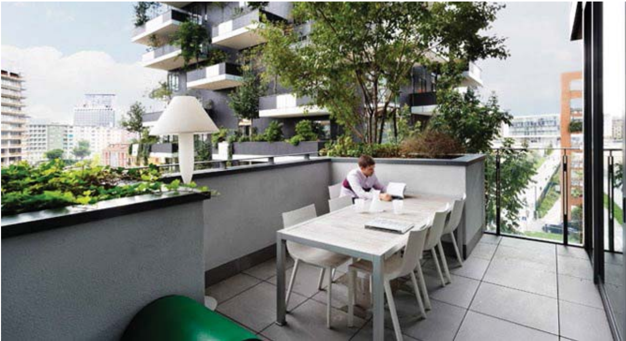
Private Terrace Planter as Divider and Parapet
