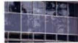
STOREFRONT TO TRANSLUCENT SPANDREL PANEL
