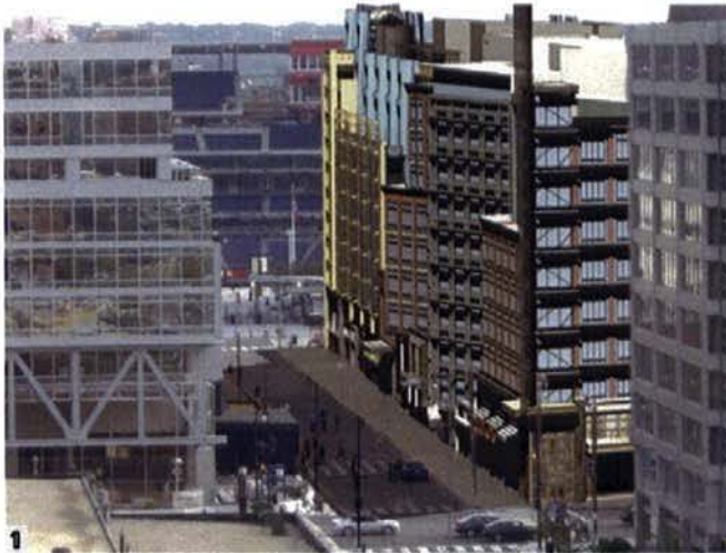
VIEW OF THE PROJECT TOWARDS THE BALLPARK
