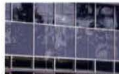
02 STOREFRONT W/ TRANSLUCENT SPANDREL PANEL
