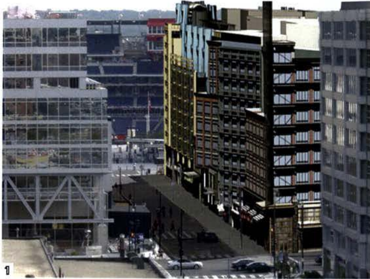
VIEW OF THE PROJECT TOWARDS THE BALLPARK
