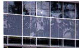
02 STOREFRONT W/ TRANSLUCENT SPANDREL PANEL
