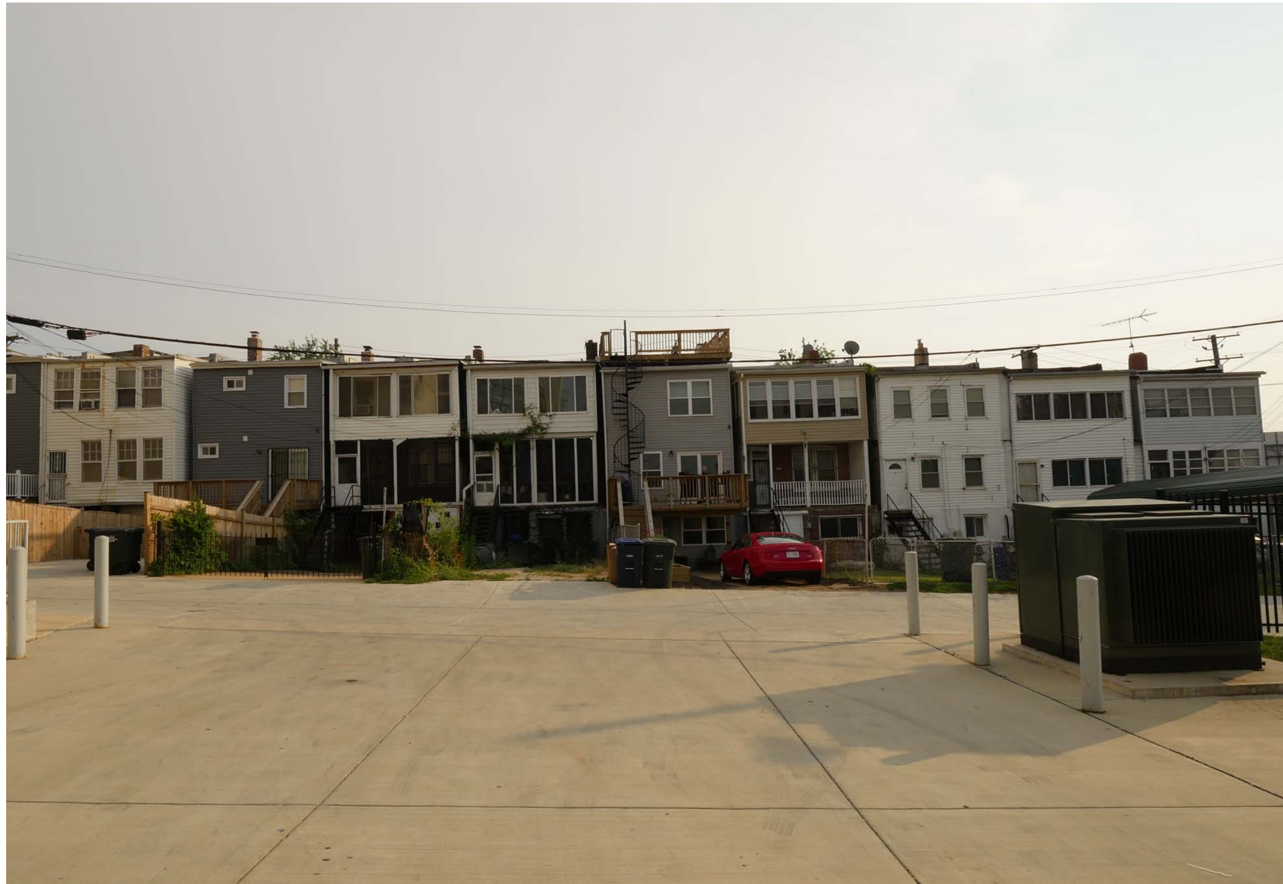
EXISTING CONDITION LOOKING SOUTH FROM EXISTING SERVICE YARD ON SITE
