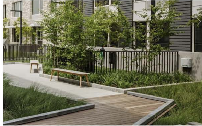
BOARDWALK OVER BIORETENTION
