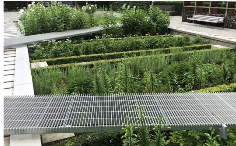
BOARDWALK OVER BIORETENTION
