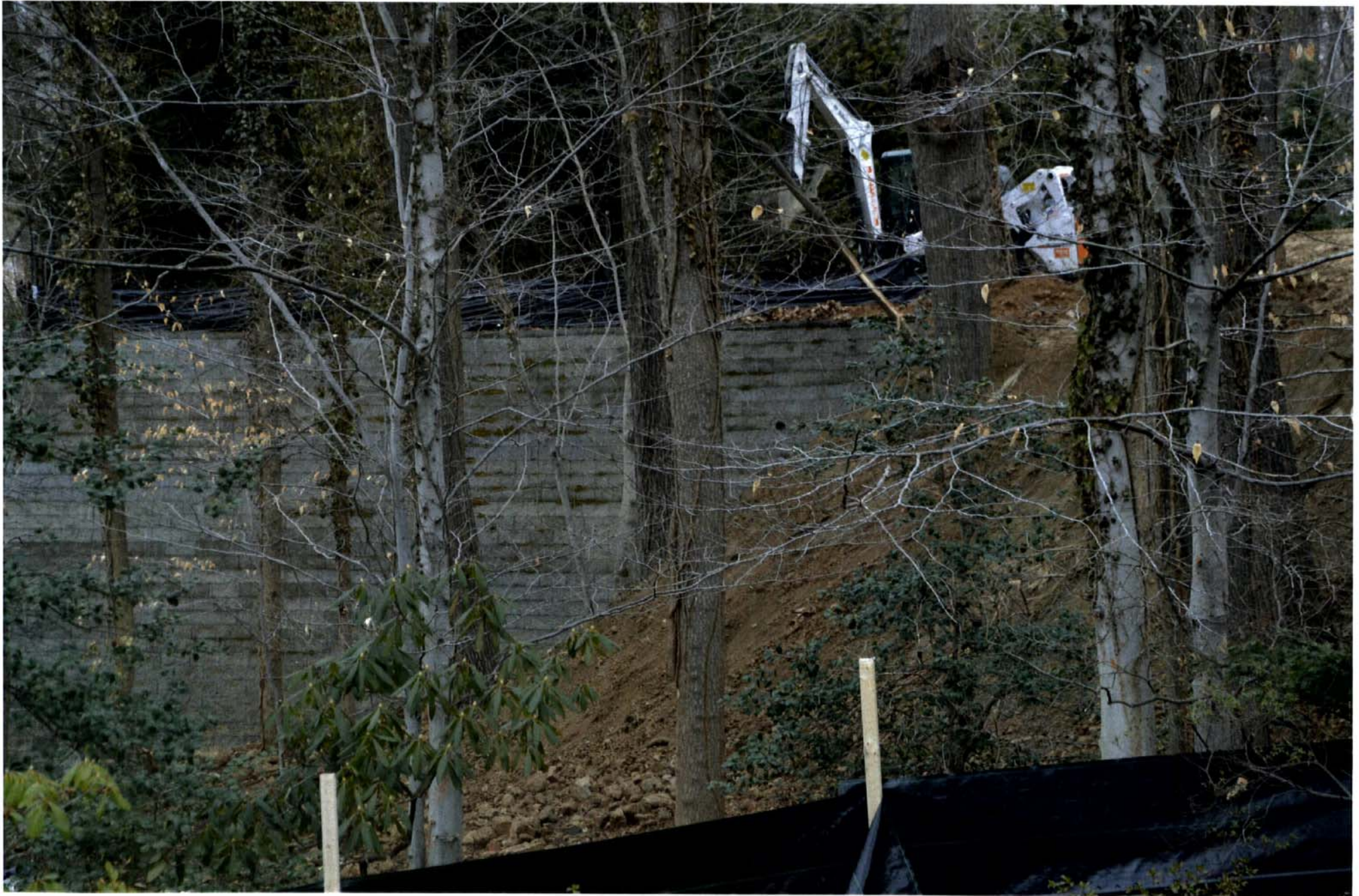
4833 Dexter Terrace, foreground. 4825 Dexter Terrace at and beyond wall. March 29, 2014.
