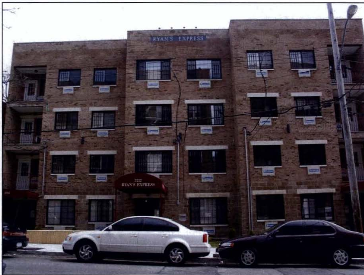
Figure 9: Recent R6 Development Using Waiver
