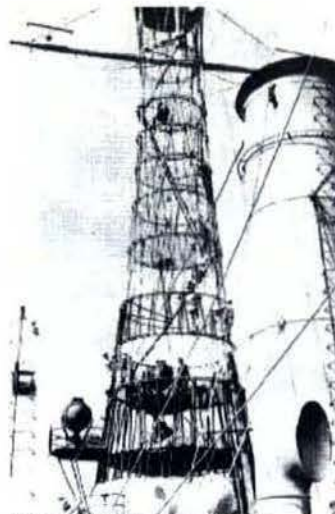
Detail of Historic Mast Structure
