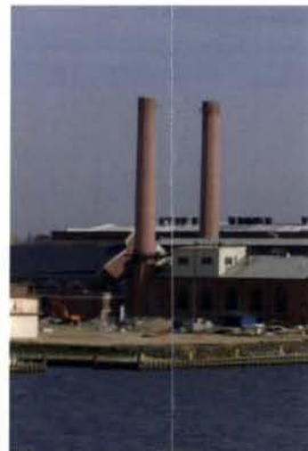
Detail of Historic Mast Structure
