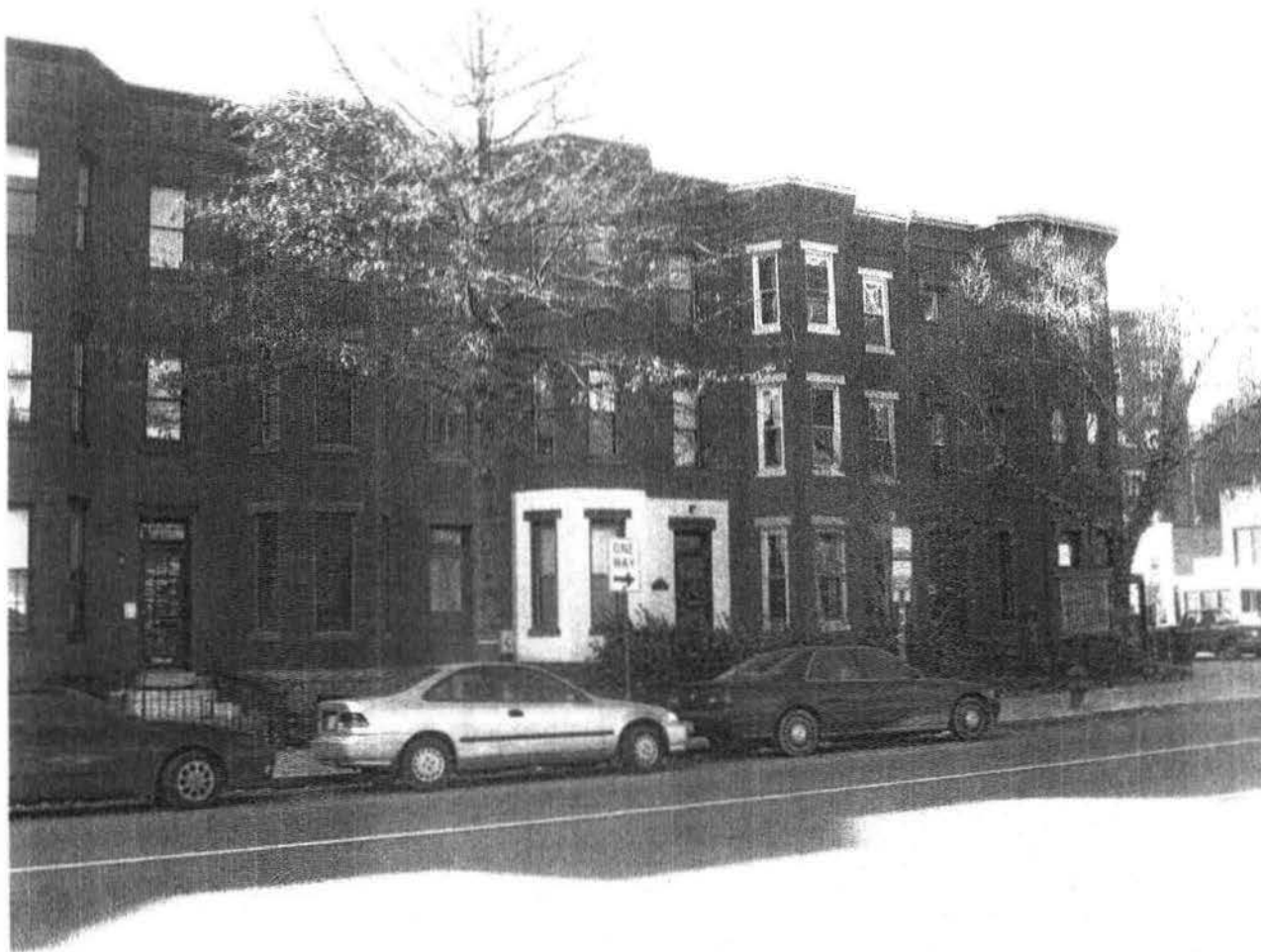
15 th Street, NW, 1900 Blk., West Side (at U Street)
