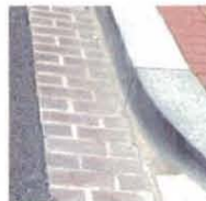
Granite Curb and Brick Gutter
