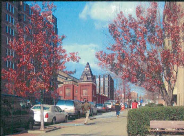
MARKET BUILDING - VIEW NORTH
