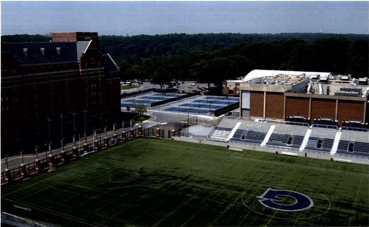
EAST VIEW OF SITE
