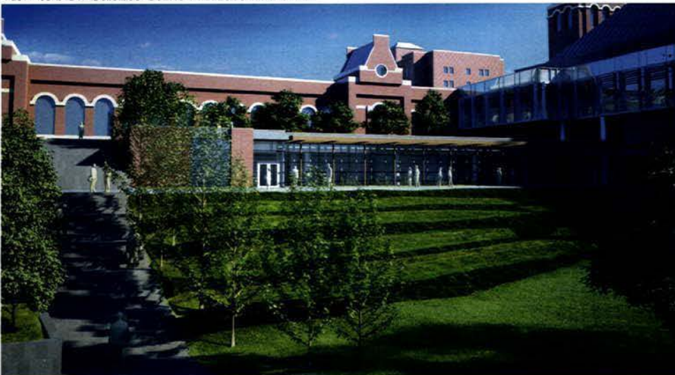
View to New Science Center Terrace and Stair
