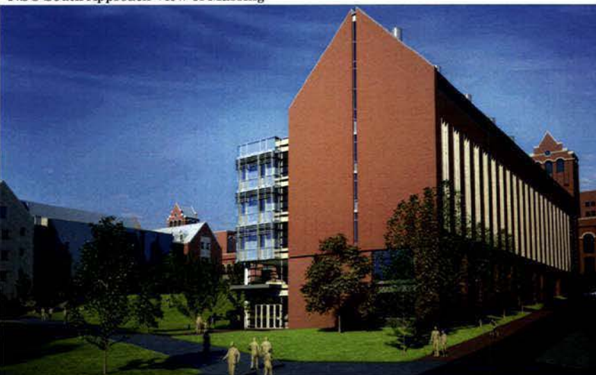
NSC South Approach View of Massing
