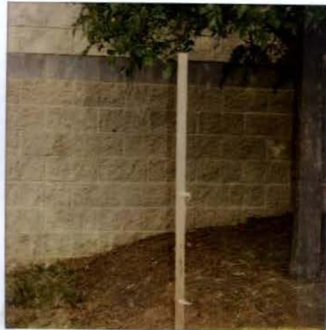
2C 07-14A 8/24/07 signs have been torn down along Brenwood Road NE site (2)
