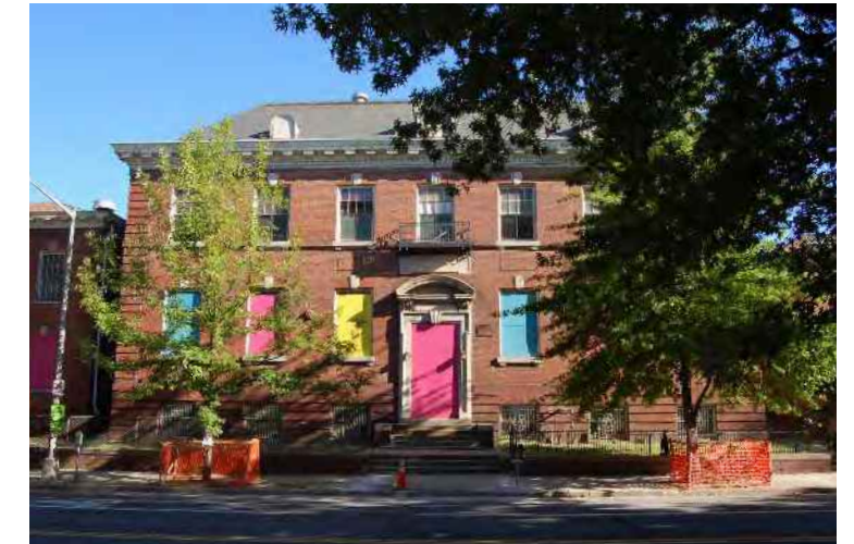
SOUTH ELEVATION (EXISTING CONDITIONS)
