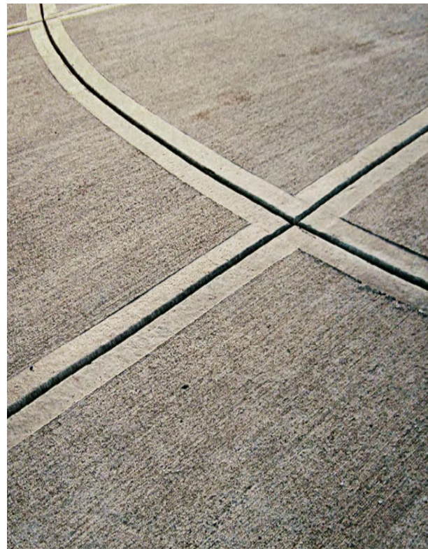
CONCRETE SIDEWALK: 3'x3' Scoring, Hairbroom Finish
