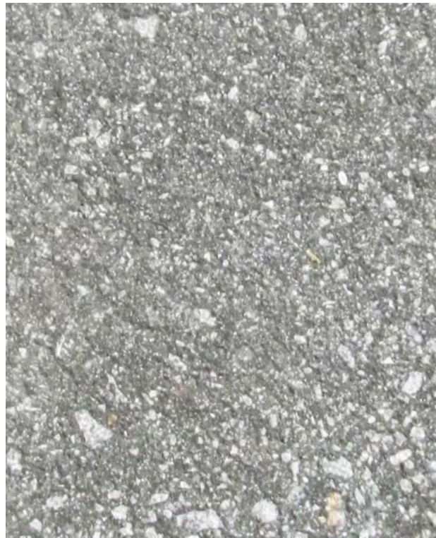
CONCRETE PAVERS, MUSEUM LOADING ZONE
