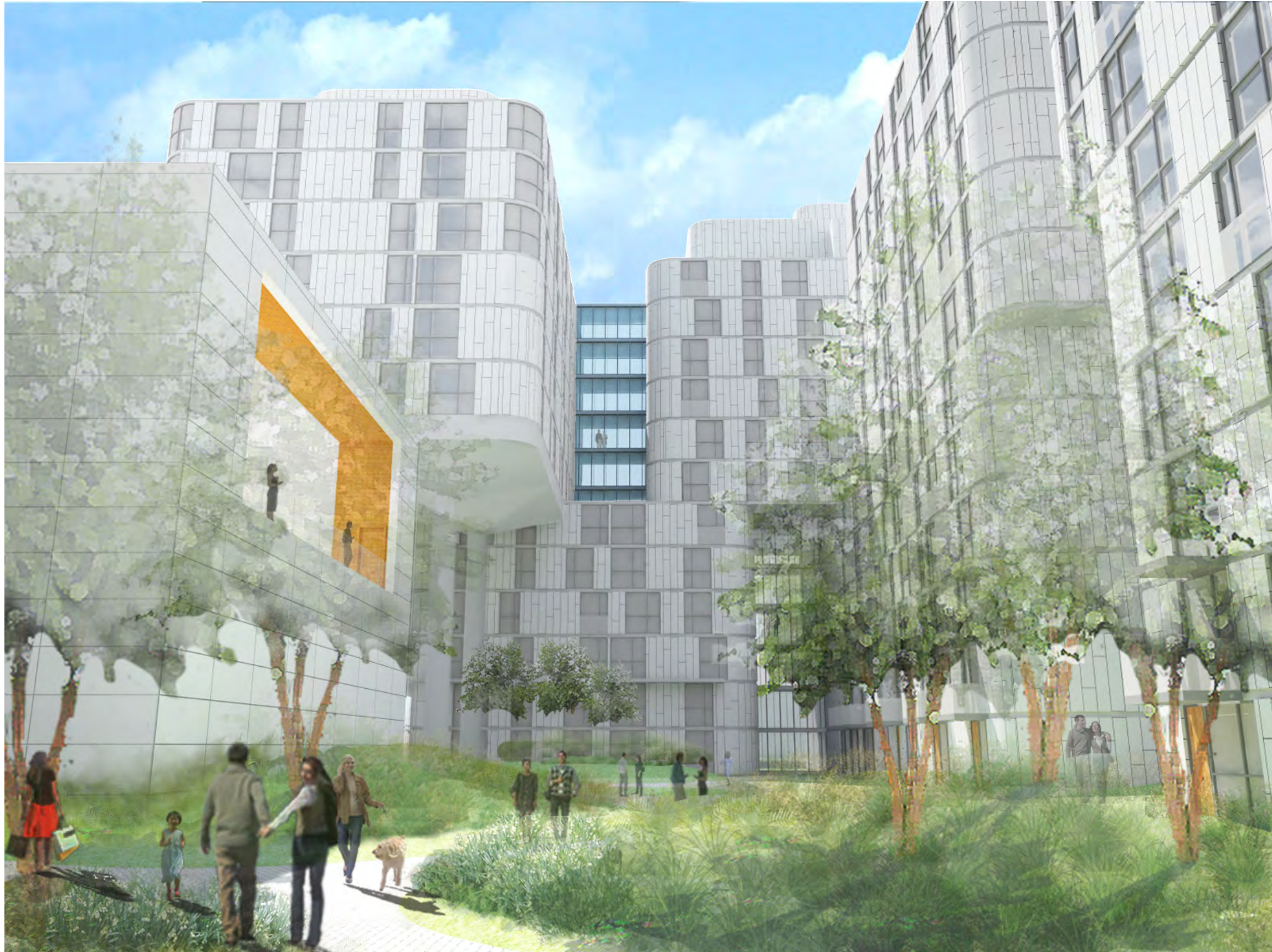
VIEW LOOKING WEST IN COURTYARD
