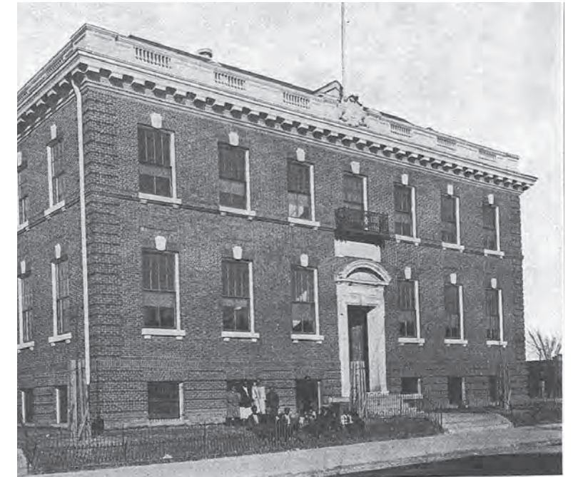
CENTRAL BUILDING PHOTOGRAPH (1908)- ROLLED CURB
