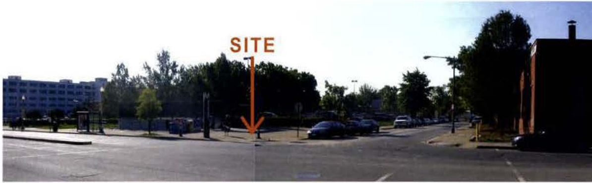
1. M & HALF STREETS INTERSECTION LOOKING SOUTH
