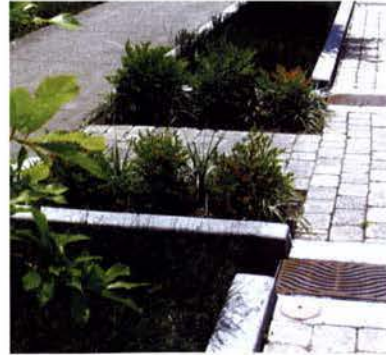
Stormwater Detention Area
