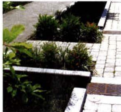
Stormwater Detention Area
