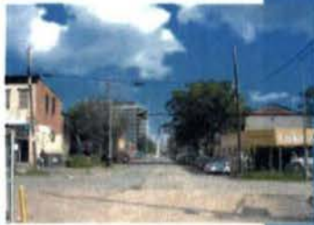
EXISTING OFFICE BUILDING UNDER CONSTRUCTION ON M STREET
