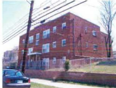
2. Existing Apartment Building on Valley Avenue
