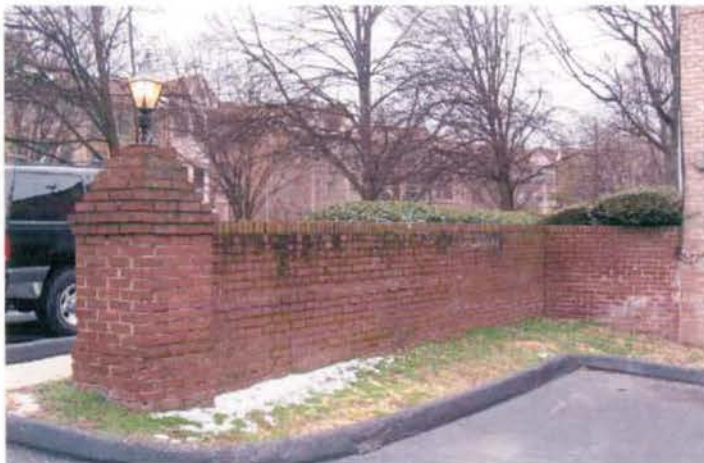
Brick Screening Walls Character
