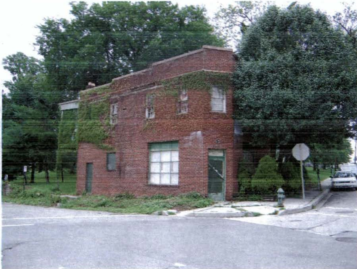
View of 4023 Chesapeake Street, N.W. from the Corner of Bell Road and Chesapeake Street
