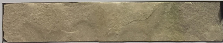
5 Stone (Florida Ave. - Ground Floor Base)
