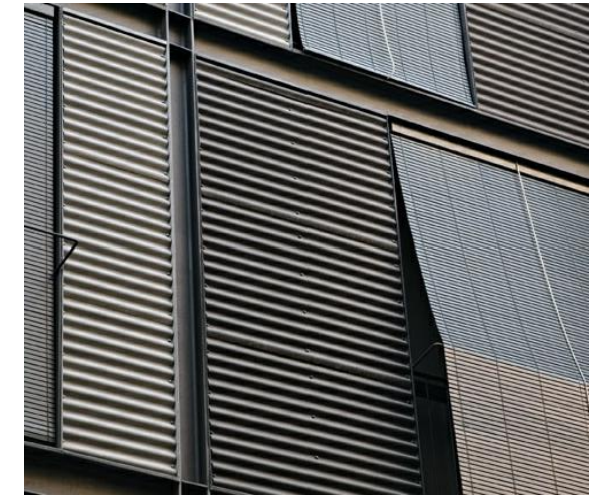
Example of Corrugated Metal Panels
