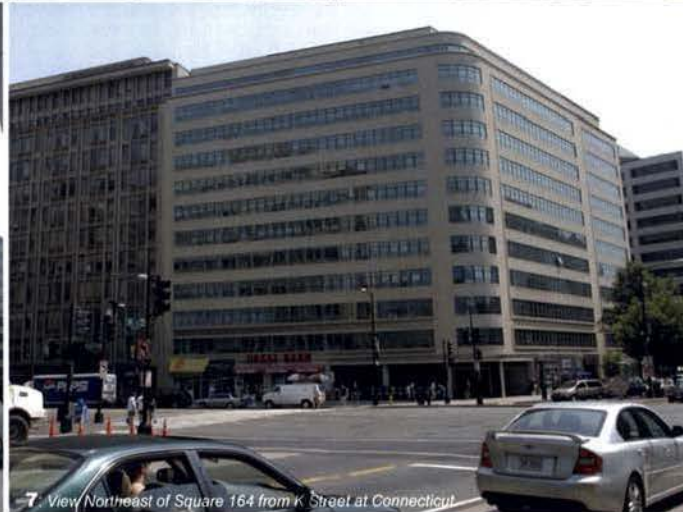
7 View Northeast of Square 164 from K Street at Connecticut
