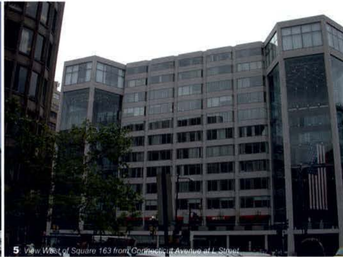
5 View West of Square 163 from Connecticut Avenue at L Street
