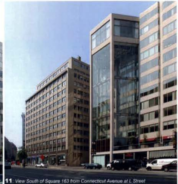
11 View South of Square 163 from Connecticut Avenue at L Street
