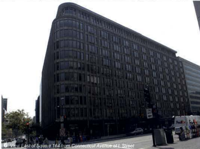
6 View East of Square 164 from Connecticut Avenue at L Street
