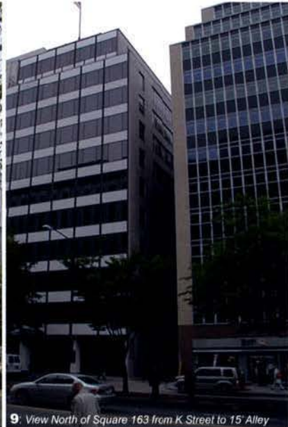
9: View North of Square 163 from K Street to 15 Alley
