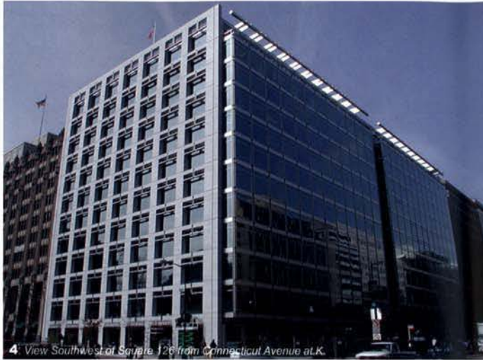
4 View Southwest of Square 126 from Connecticut Avenue at K Street
