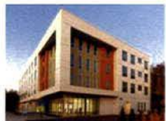
Brookland Artspace Lofts
