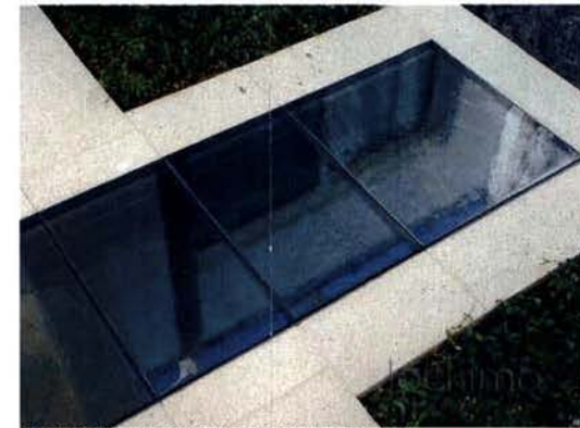
AREAWAY, STRUCTURAL GLASS ROOF
