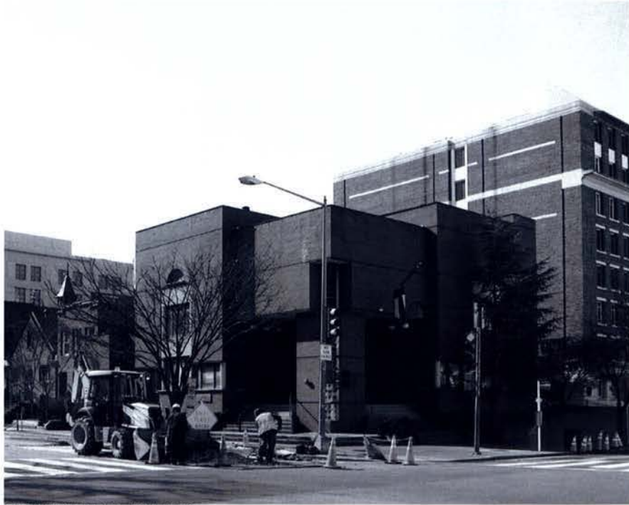
EXISTING HILLEL BUILDING
