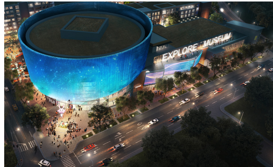
CONNECT PLAZA & METRO STATION
