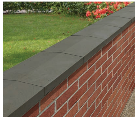
MASONRY PLANTER WALLS
