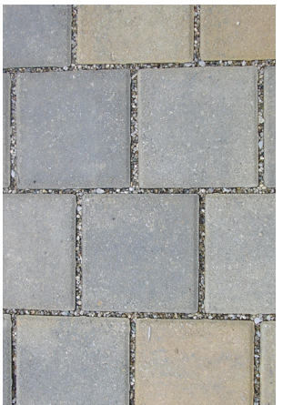
PERMEABLE UNIT PAVERS
