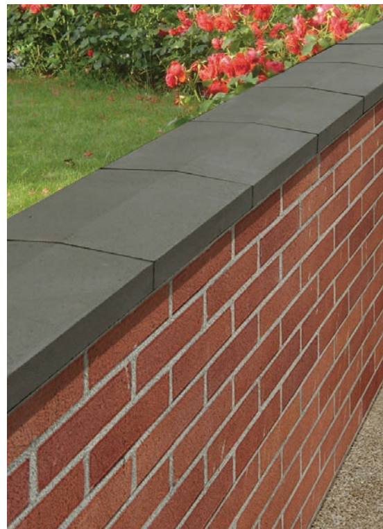
BRICK PLANTER WALL
