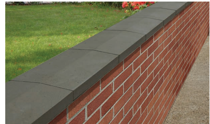
MASONRY PLANTER WALL
