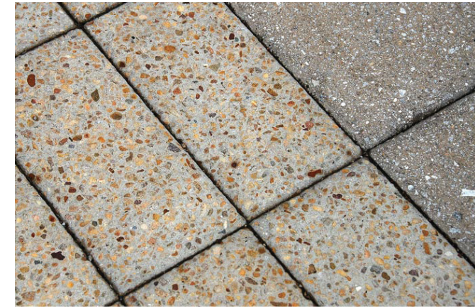
PRECAST UNIT PAVERS AT ENTRY
