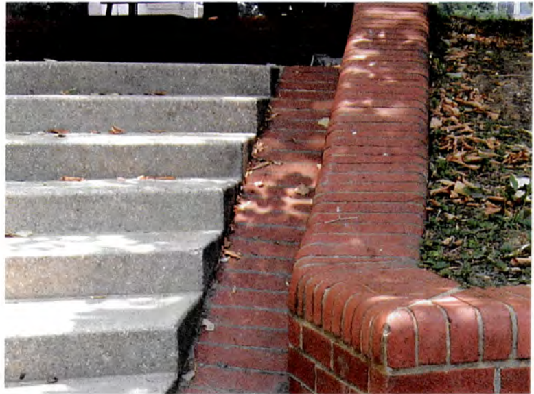
Figure 1 Brick runnel and concrete steps
