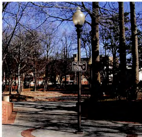
Figure 10 Current pole-mounted lights
