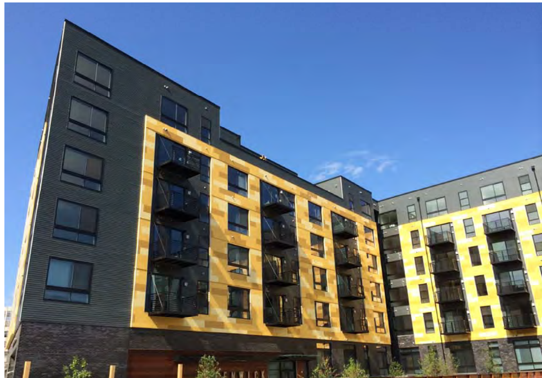
3. FENWICK STATION: SILVER SPRING, VA MATERIAL: PAINTED SMOOTH FIBER-CEMENT SIDING (BACKGROUND PLANE)
