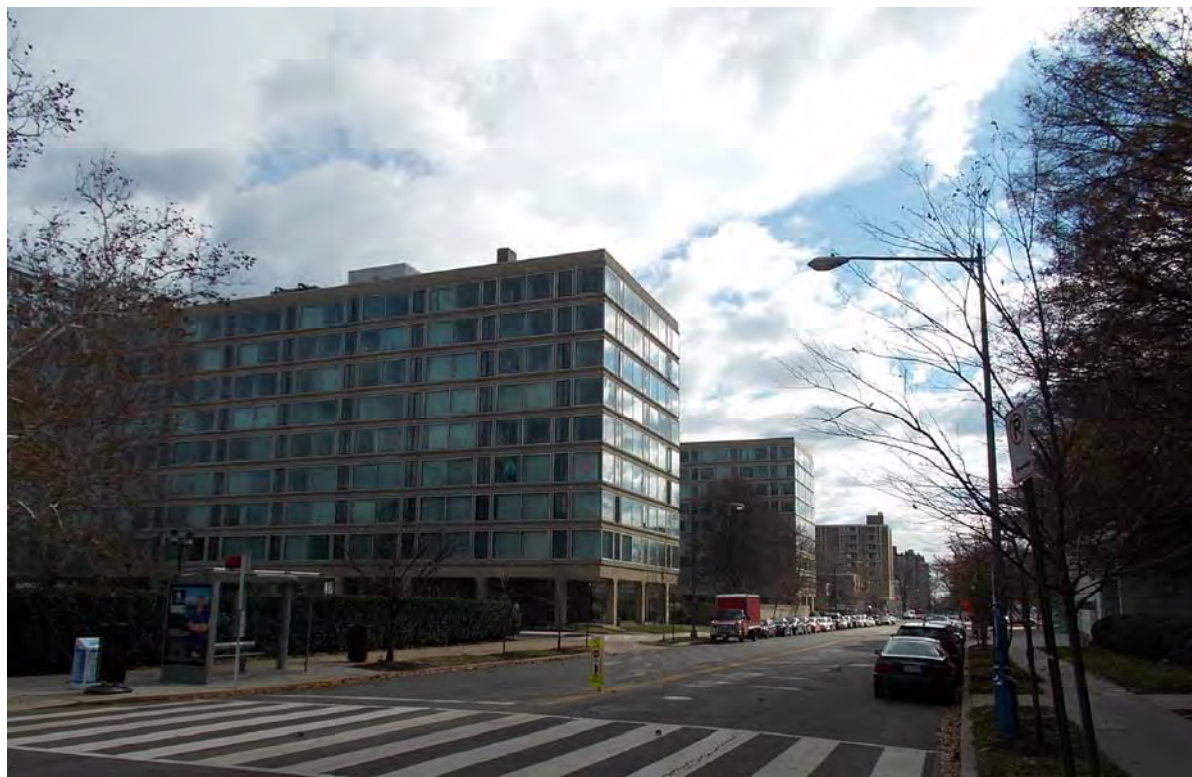
6 VIEW OF 6TH STREET LOOKING SOUTH
