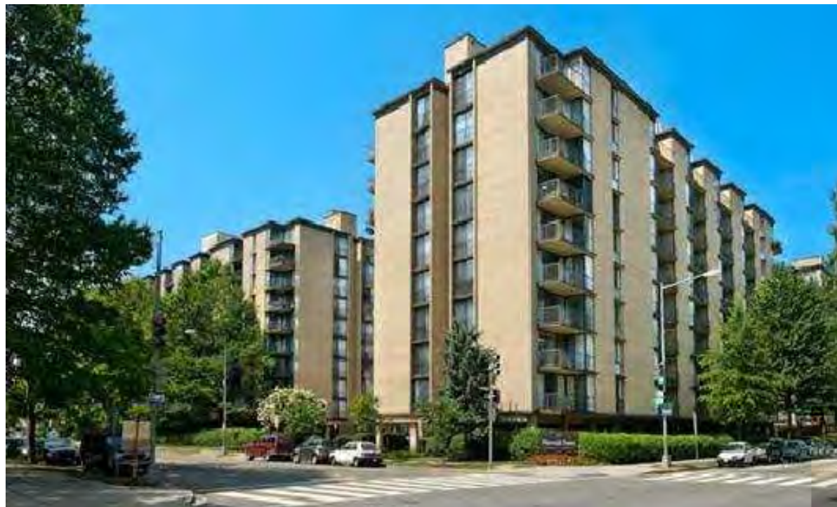
12 WATERSIDE APARTMENTS TO WEST OF SITE
