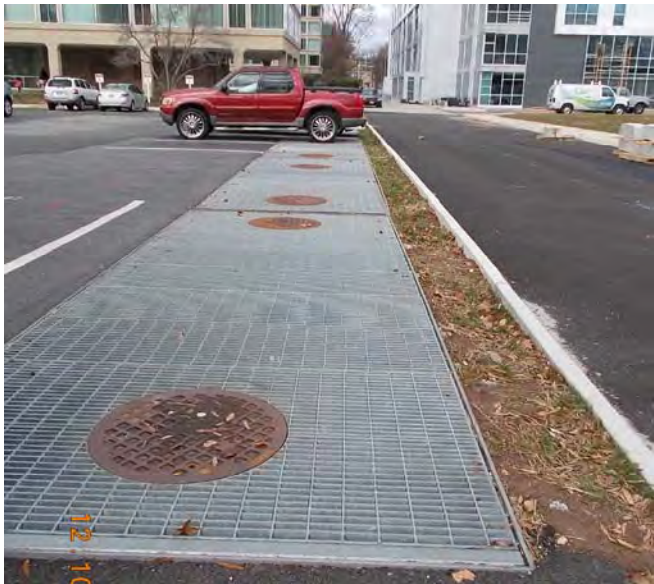
3 EASEMENT WEST OF ALLEY LOOKING NORTH
