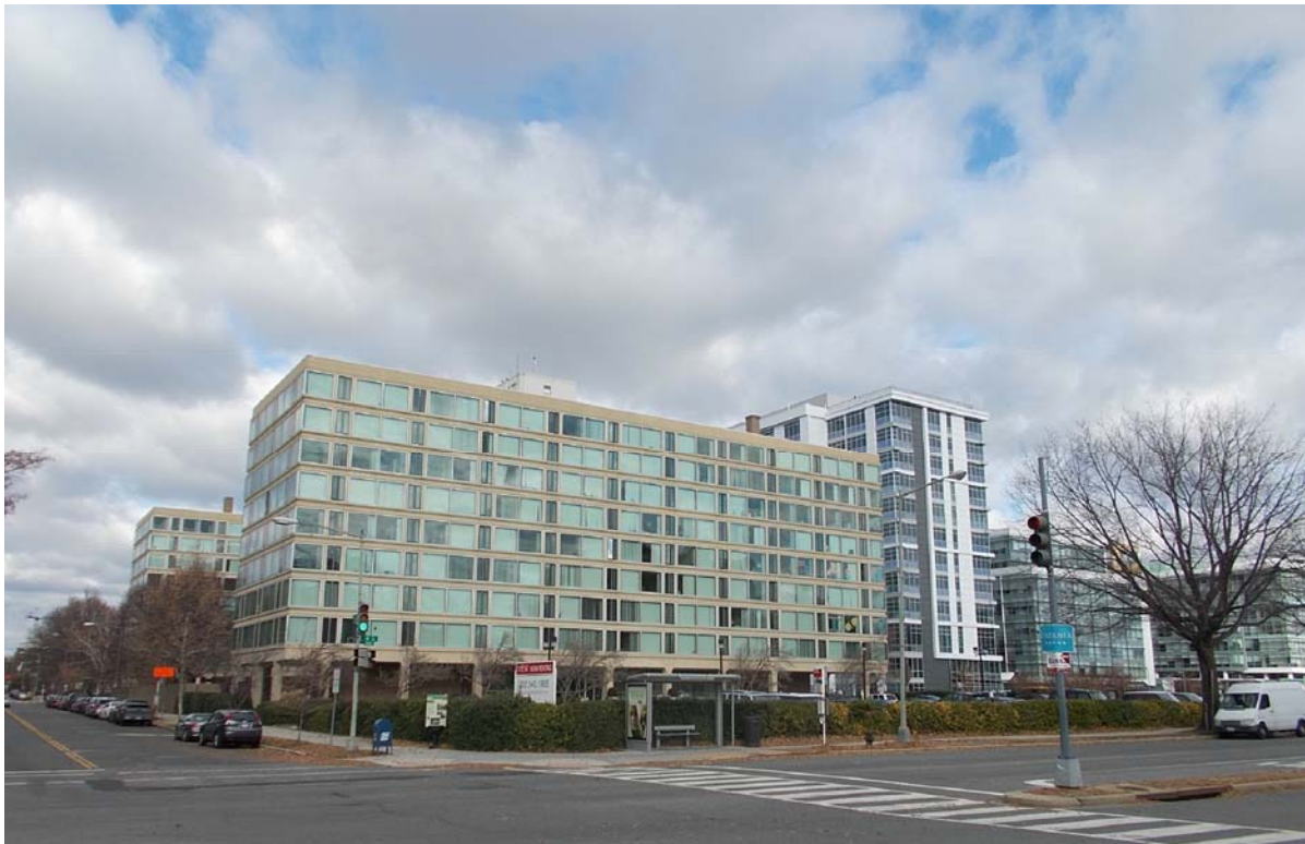
7 VIEW OF M STREET LOOKING EAST
