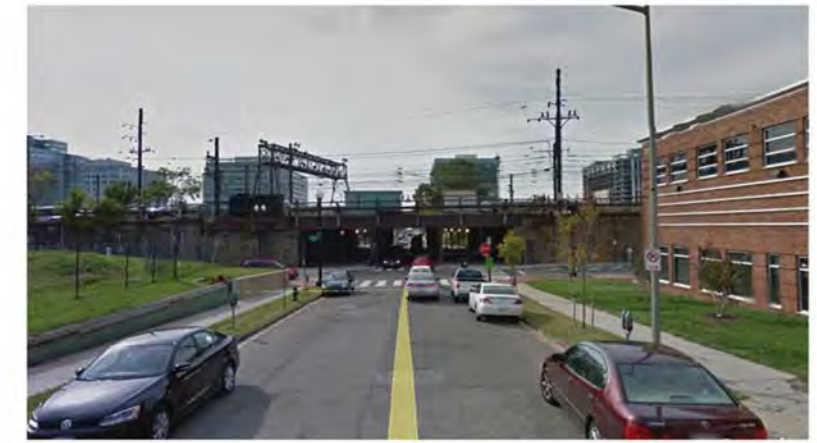
4 L STREET - VIEW WEST
