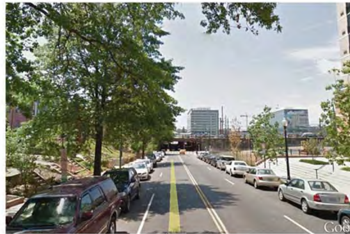
9 K STREET OVERPASS - VIEW WEST
