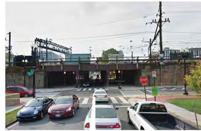
3 L STREET OVERPASS - VIEW WEST
