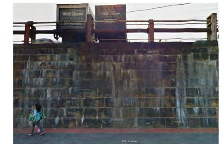
14 2ND STREET- WALL
