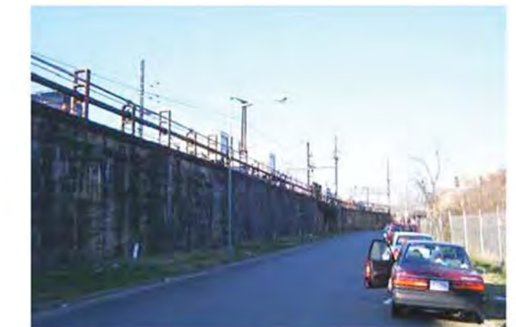
12 2ND STREET - VIEW NORTH
