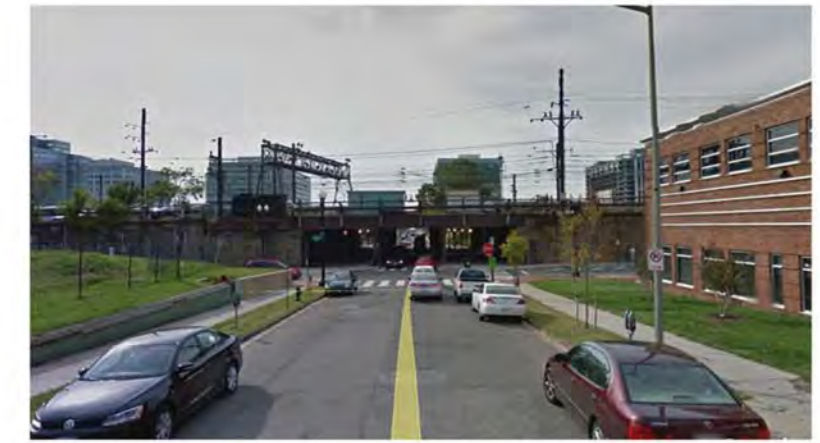
4 L STREET - VIEW WEST
