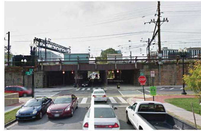
3 L STREET OVERPASS - VIEW WEST
