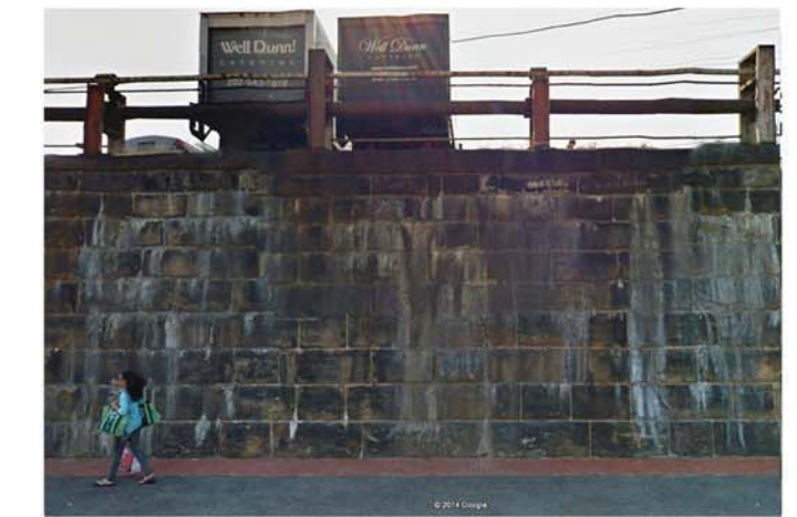
14 2ND STREET- WALL
