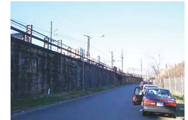
12 2ND STREET - VIEW NORTH
