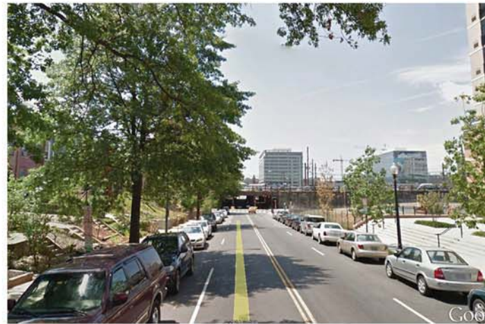
9 K STREET OVERPASS - VIEW WEST
