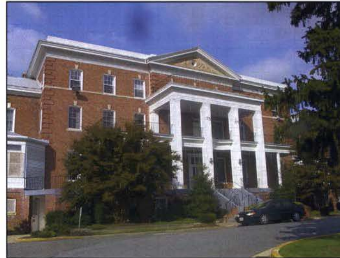
View of Existing Building, proposed to be Main Condo Building
