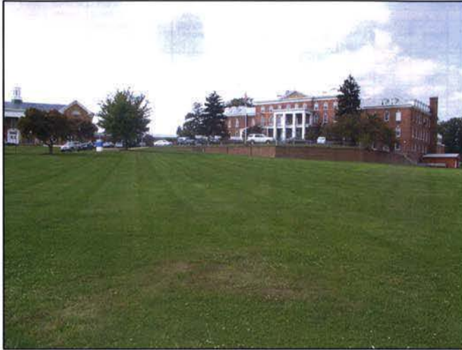
View looking North from intersection of New Hampshire Avenue and Peabody Street
