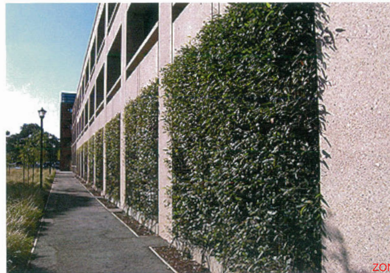
Example of Parking Garage Green Screen – Stanford University
